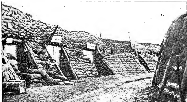
PROTECTED SHELTERS FOR AMBULANCE WORK IN CHAMPAGNE
